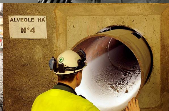
HLW-cell excavation test
