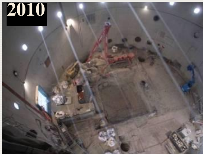
Big internal structures demolished
