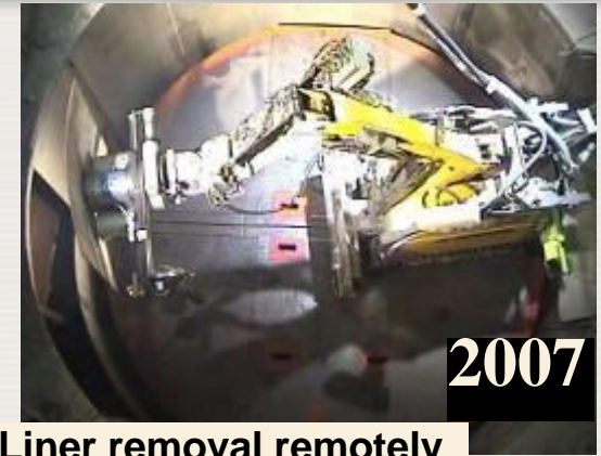
Liner removal remotely
