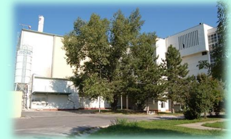
RAW Treatment and Conditioning Facilities
