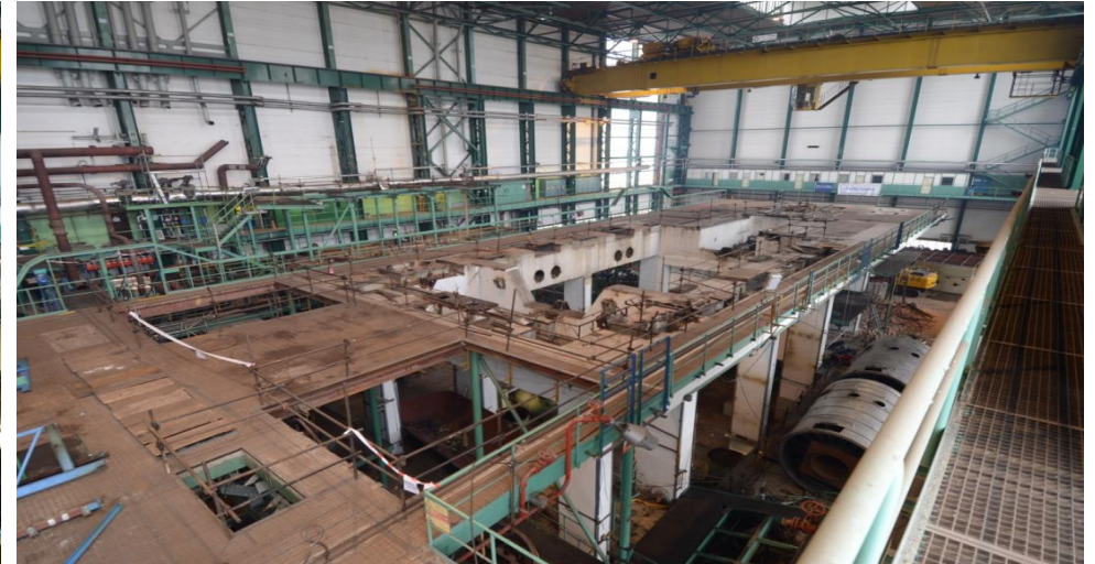
TG 22 after dismantling
