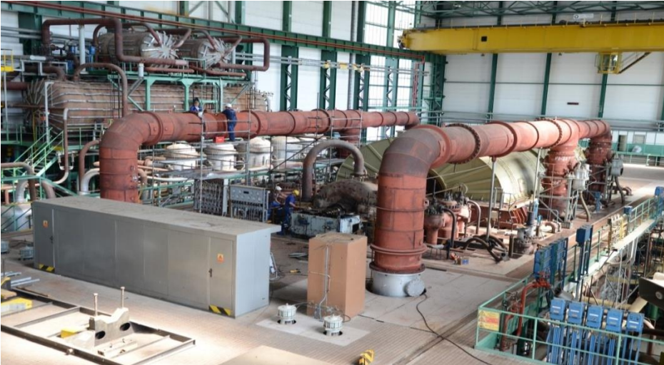
TG 22 before dismantling
