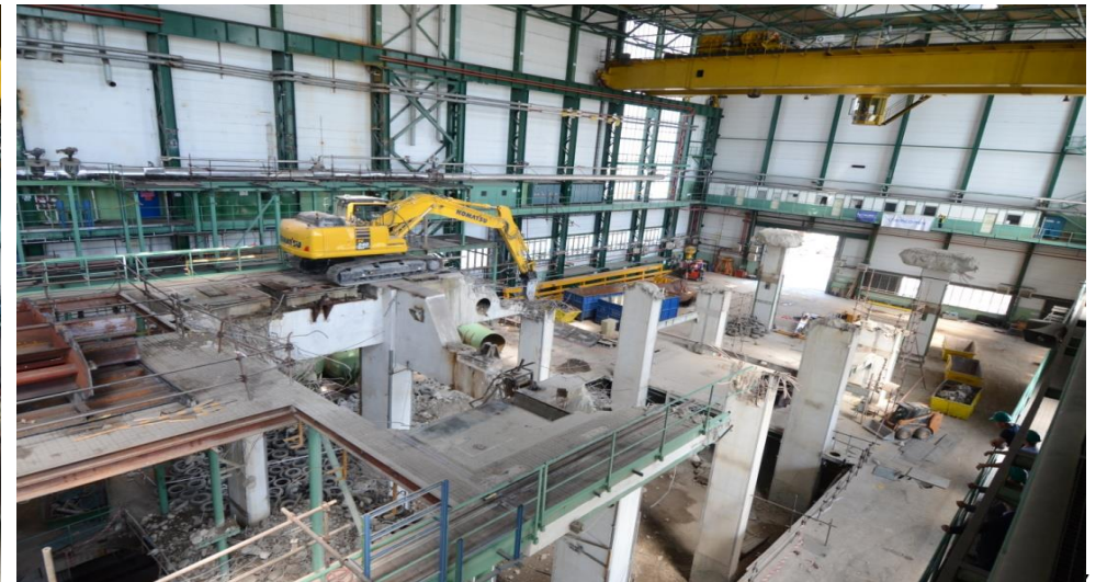
TG 22 support construction after
